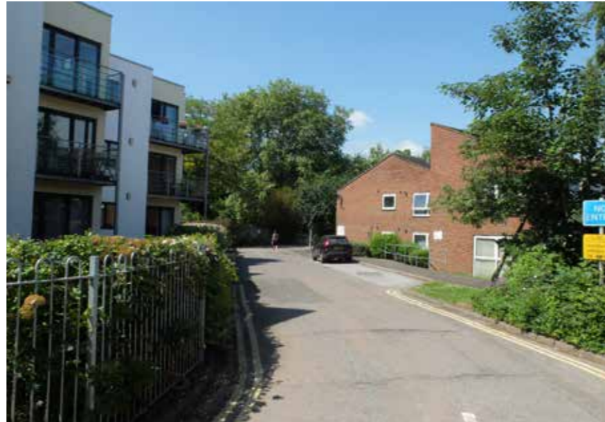
1) site seen from the south
