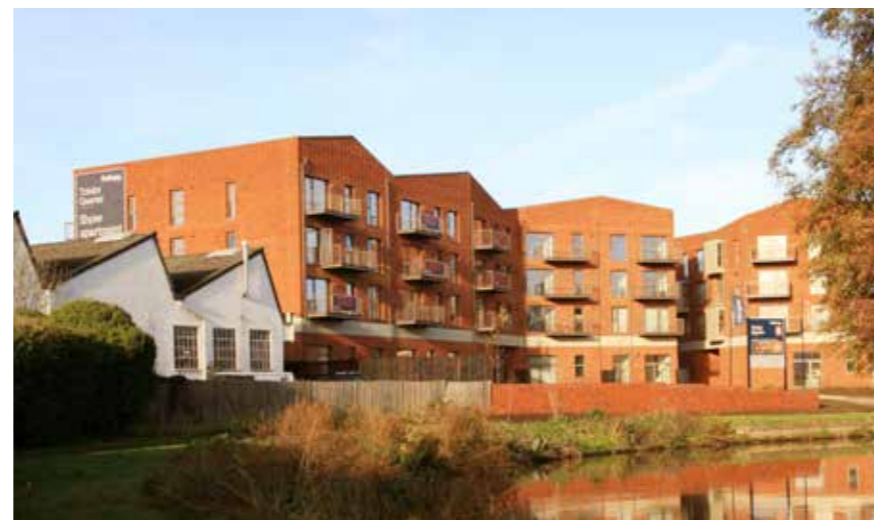
Walnut Tree Close, Guildford - FBM Architects
