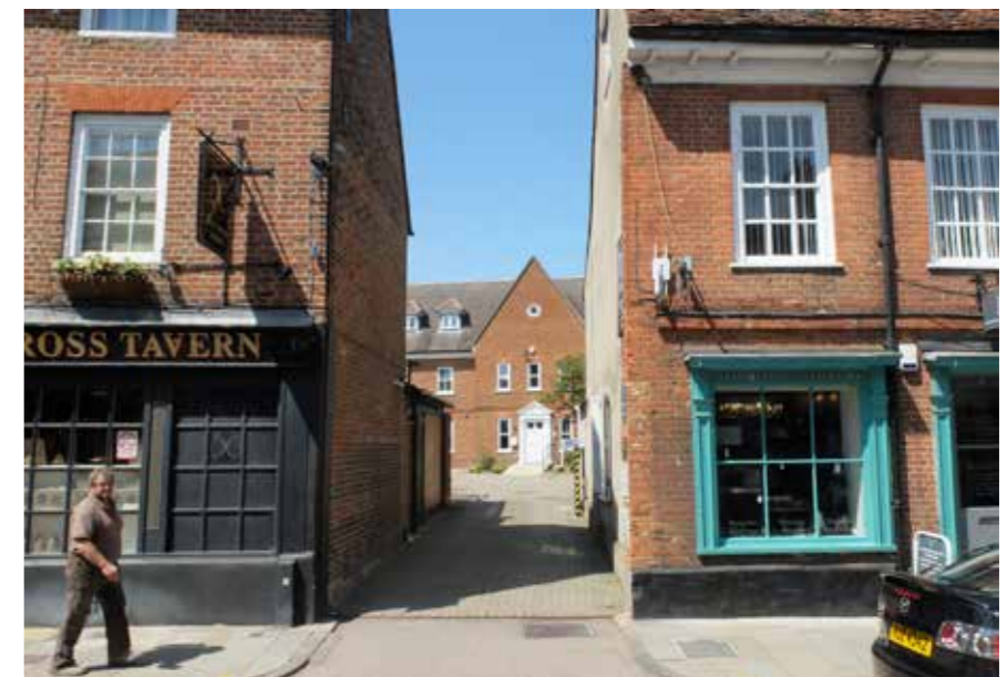
4 Office building access off the high street
