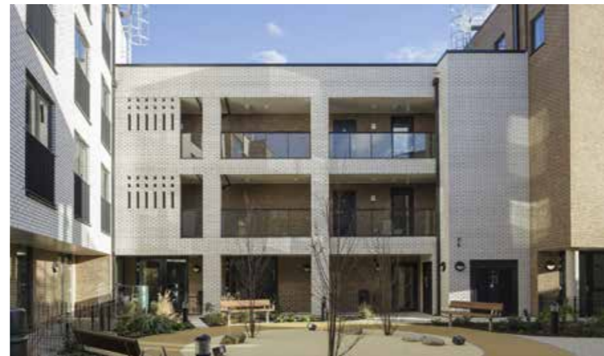
Salcombe Road, Hackney - FBM Architects
