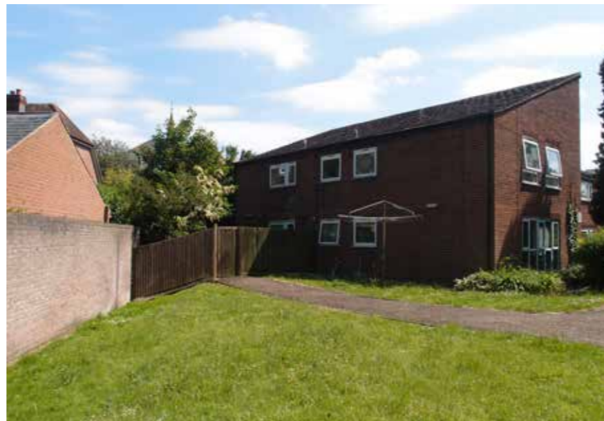
2) The site seen from north-east
